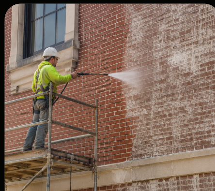
MASONRY CLEANING
