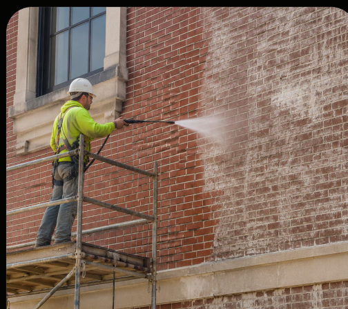
MASONRY CLEANING
